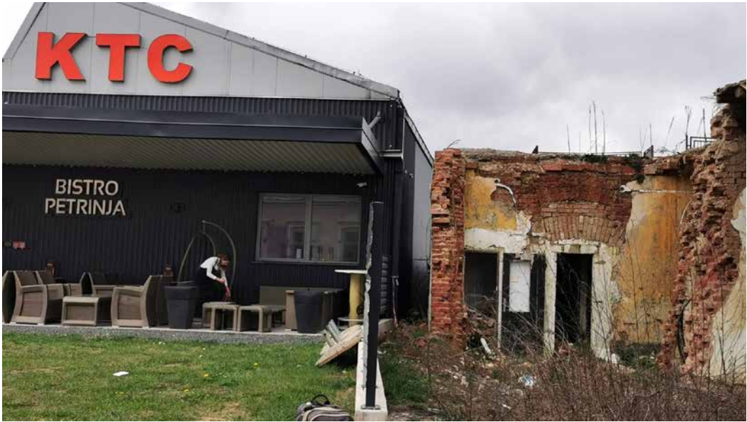
FIGURE 3. Two faces of post-earthquake Petrinja: a ruined house on the right and a container-like structure on the left (March 2023, photo credit: Dan Podjed).
