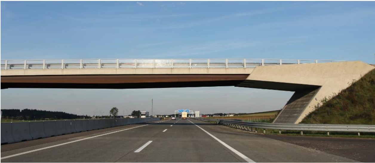
Fig 5:. Construction of Motorways has to deal with building culture
