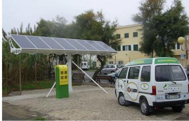
Figure 5: The integrated photovoltaic charging station
