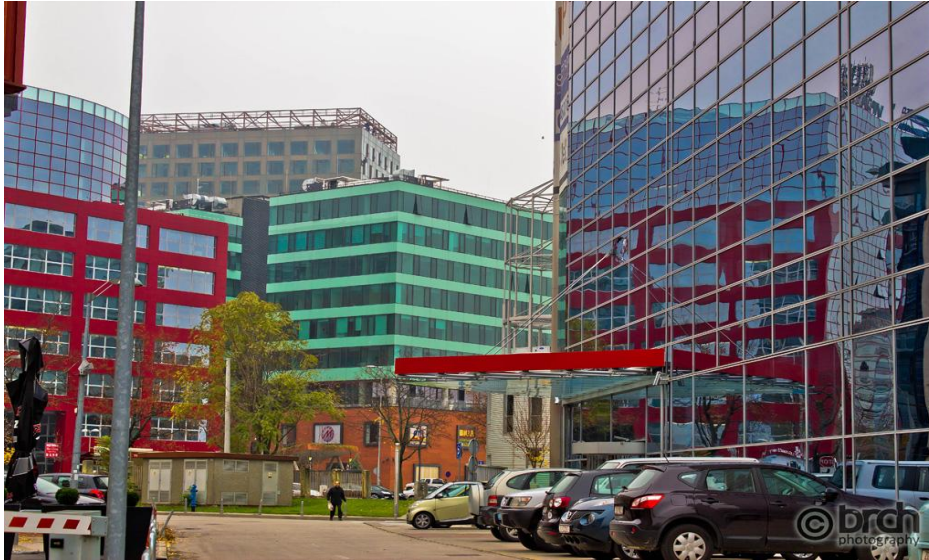
Picture 3 High density housing in a business district
