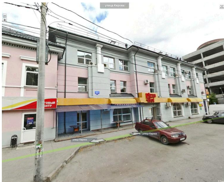
Fig.4 Façade of building, Kirov street.
